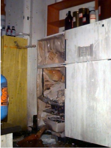
Doors ripped off unit
